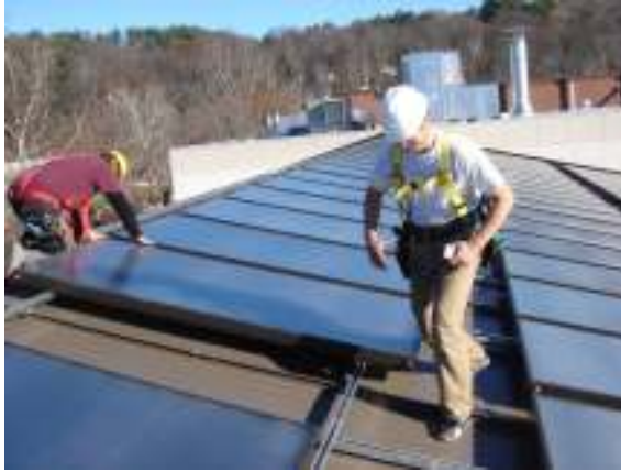
Southern VT Recreation Center, Springfield VT 130 kW thermal array saves $15,000 a year in fuel
