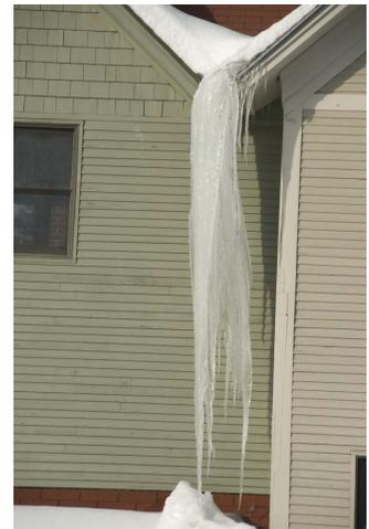
*Figure 1: Icicles like this are a good indication of poorly performing insulation and/ or ventilation.*
