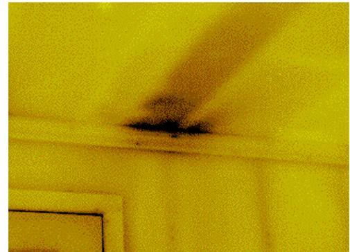
Figure 5: Batt insulation is susceptible to air infiltration. The fiberglass shown here does not stop airflow directly into the home or indirectly into the ceiling section.
