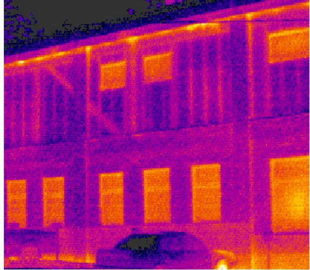
*Figure 6: All the framing and insulation is clearly visible in this apartment building. Pressure differences in the building, known as stack effect, result in air leaking past the envelope through various pathways and exiting out near the top plate of the wall. The fiberglass batt insulation does little to slow the movement of air.*
