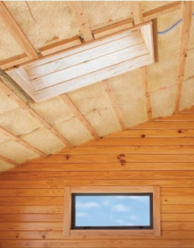
▲ **GACO WESTERN.** HFC-blown WallFoam 184 BIO open-cell spray-foam insulation is derived from naturally renewable oils, post-consumer recycled plastics, and pre-consumer recycled materials. The Class I fire-rated foam offers an average R-value of 6.2 per inch, the firm says, and can reduce a home's carbon footprint by up to 13% a year, the company claims. 877.699.4226. www.gaco.com. Circle xxx.
