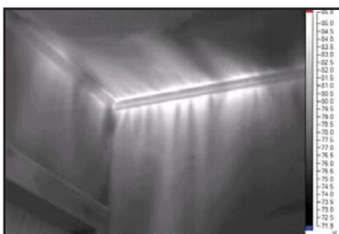
The use of a blower door helps make summer inspections possible.
