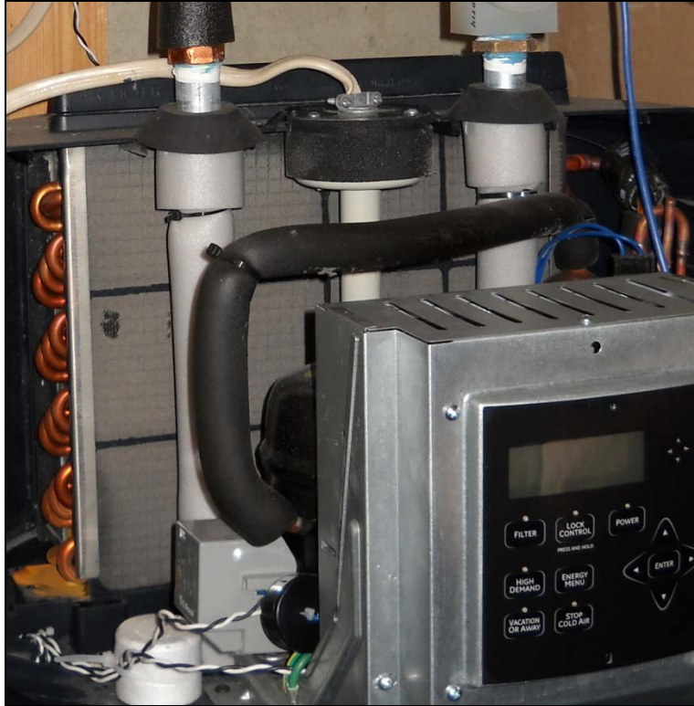
Figure 9. A filter in a HPWH that had not been cleaned in several months. A finger mark on the left of the filter shows where dirt was rubbed away.
