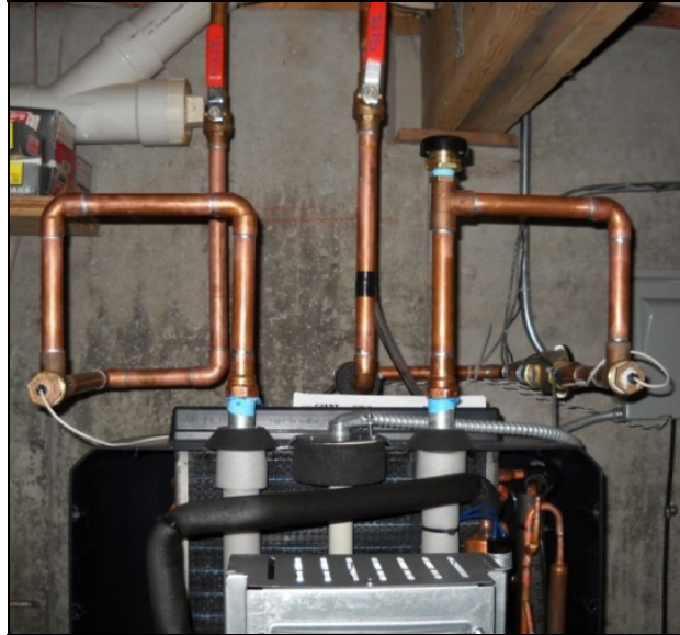
Figure 7. Water heater with heat traps. Insulation of hot water lines is also recommended.
